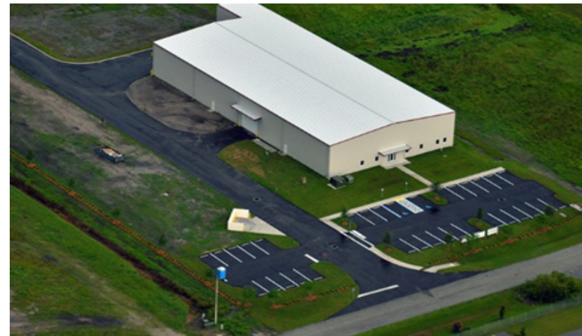
Fig. 4.10 Industrial Development in Hardee County's Commerce Park
