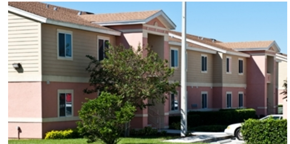
Fig. 05.29 Country Walk Garden apartment building
