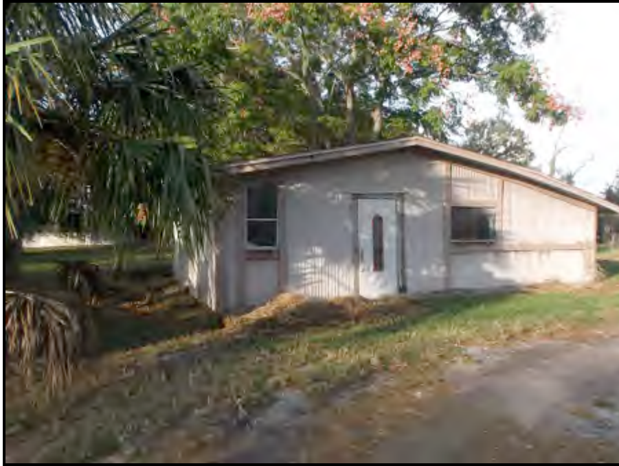
5. View of improvements at 735 5 th Avenue South, on tax parcel no. 09-34-25-0270-0000A-0006.
